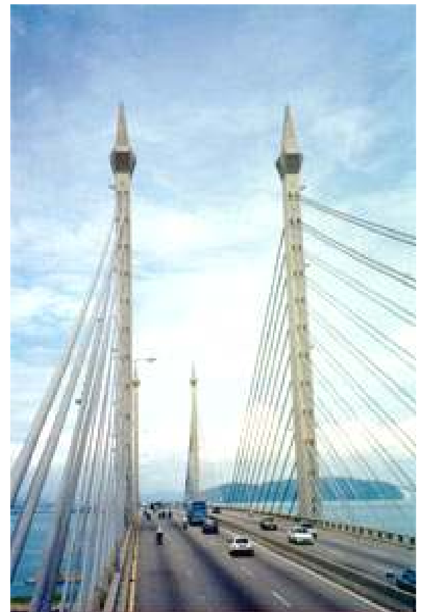
FIGURE 5: Free standing pylons topped with symbolic parasols.
