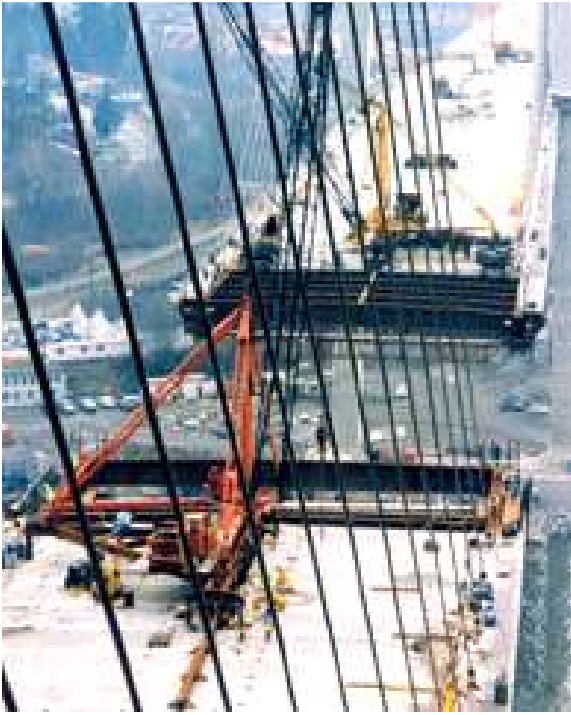
FIGURE 4: Mid-span derricks assemble steel deck framing.
