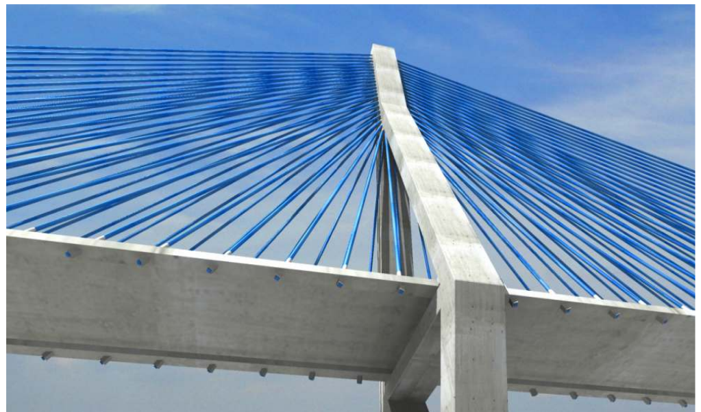
FIGURE 3: One of the twin, 315.83' towers supporting half of the 940' main-span and two side spans of 440' and 90'.
