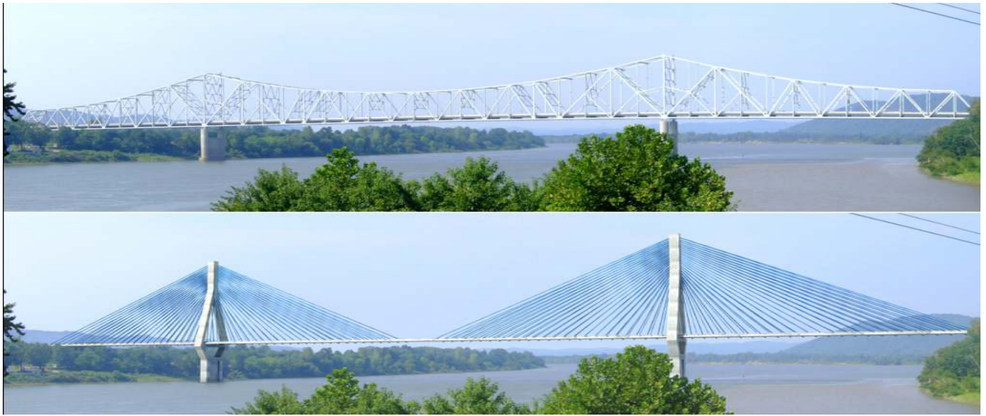
FIGURE 4: The competing designs were a study in contrasting structural schemes: top scheme features flexure; bottom, tension-compression
