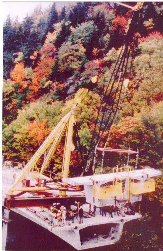
FIGURE 2: Superstructure segments delivered to and advanced from roadway deck.
