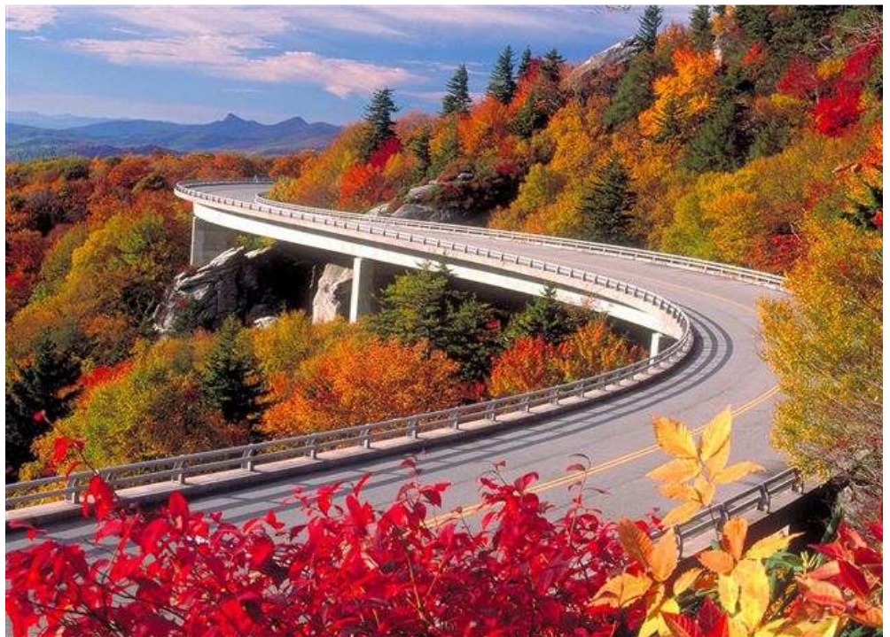
FIGURE 1: Elevated roadway hugs the east slope of Grandfather Mountain while sidestepping rock outcrops.
