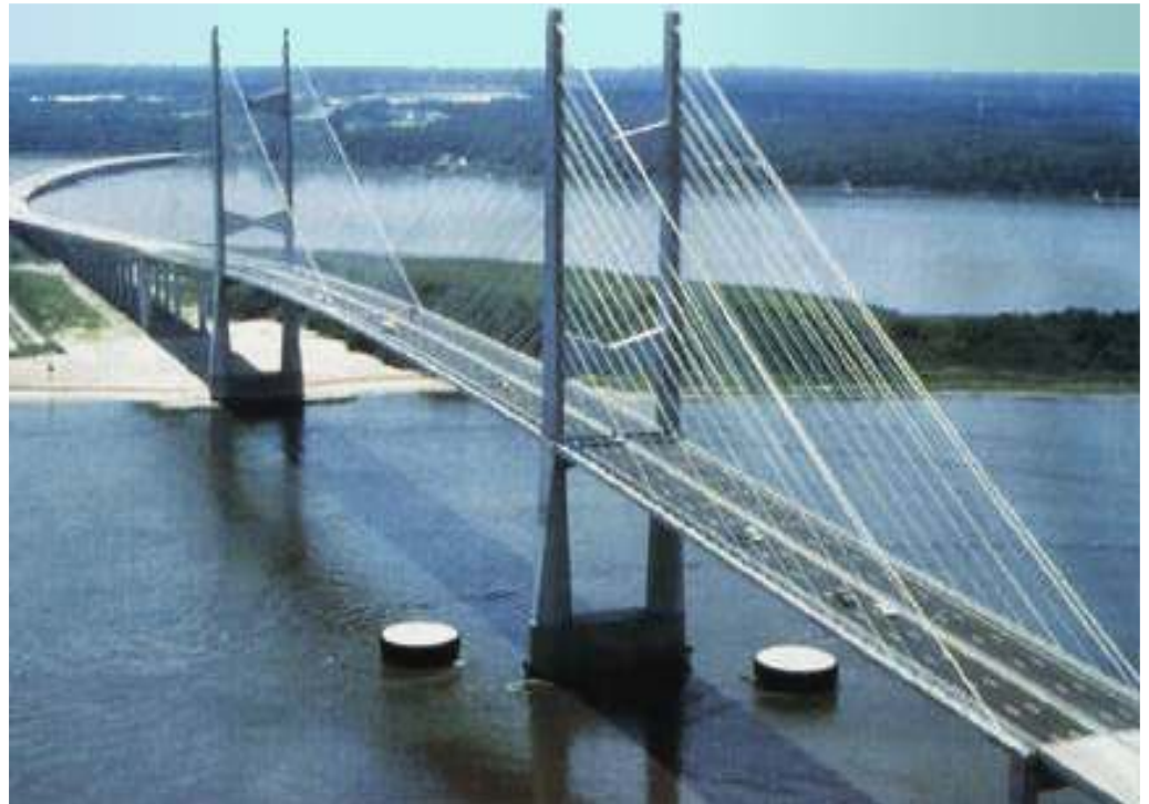
FIGURE 1: TWO SETS OF BOW-TIE TOWER STRUTS AND TWO PLANES OF HARPED TENDON STAYS (PARALLEL STAYS)
