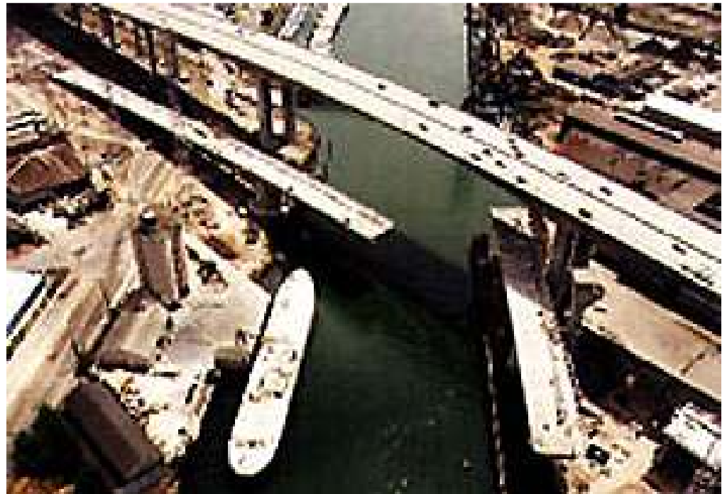
FIGURE 5: NORTH LEAF (LEFT) CLOSED, SOUTH LEAF (RIGHT) FULLY OPENED THROUGH A 45 DEGREE ARC, PARALLEL WITH THE DUWAMISH RIVER
