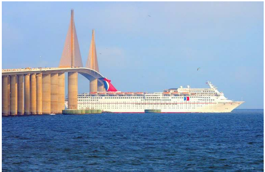
Figure 1: The 14'-8" deep, 4000' long girder spans Tampa Bay's main shipping channel.
