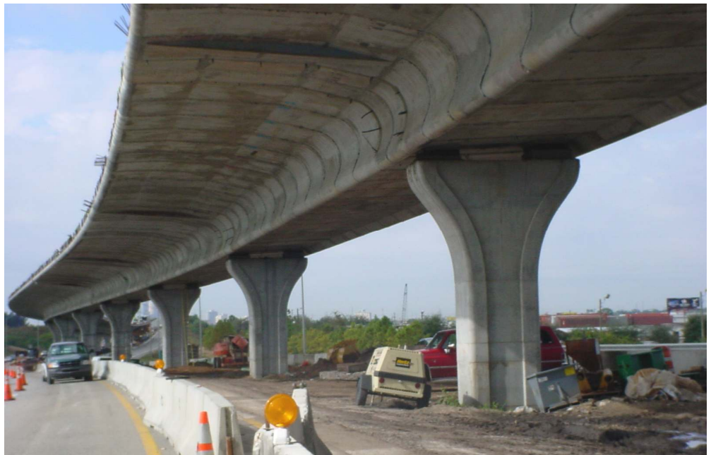
Figure 4: Superstructure with 20'+ Cantilevered Roadway Deck
