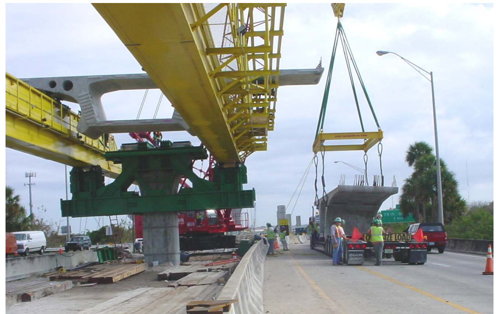
Figure 3: Erection Bracket Supporting Launching Girder
