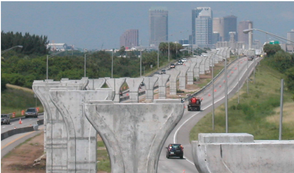
Figure 1: Cast-in-Place Substructure Anticipating Pre-Cast Superstructure
