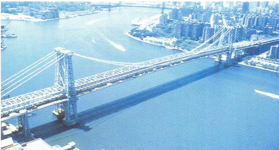
FIGURE 1: Aerial view of the Williamsburg Bridge.
