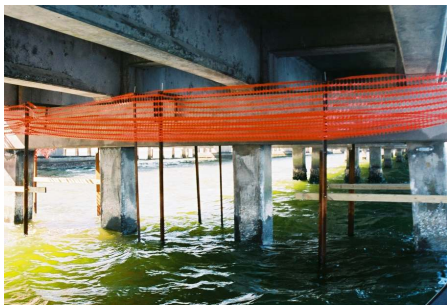
FIGURE 4: Existing piles' surface cleaned
