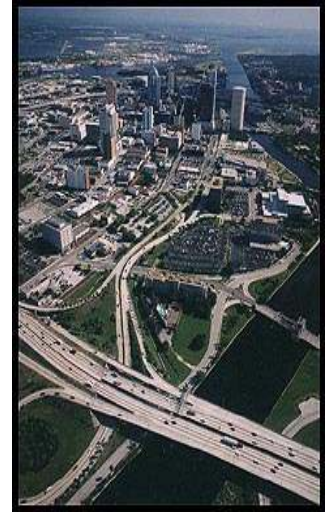
TAMPA INTERSTATE SYSTEM
