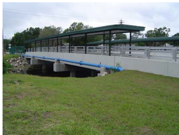
Completed Webb Road Bridge Replacement
