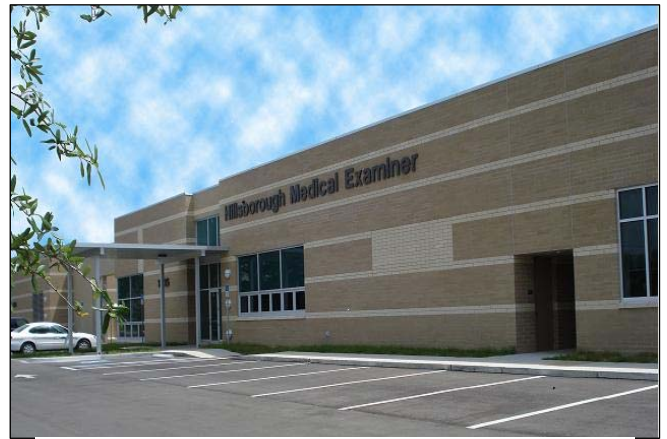
New Hillsborough County Medical Examiner Facility was completed in FY 08
