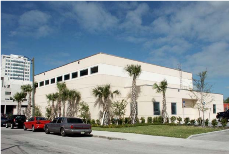
New Chiller Plant
