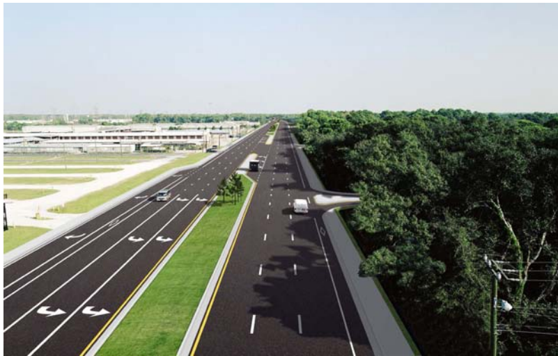
Racetrack Road (After Improvements)
