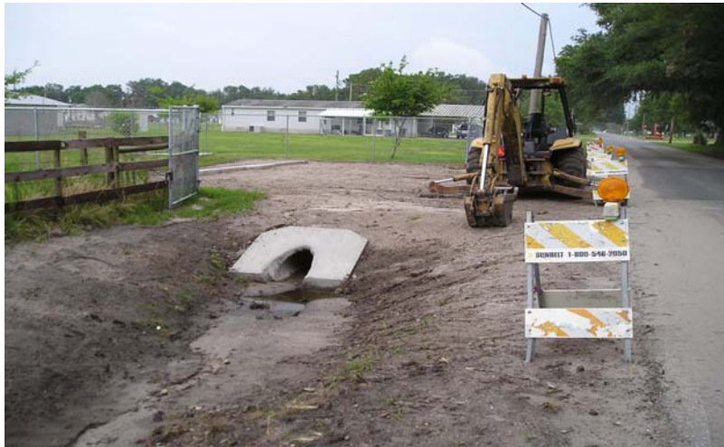
Clay Turner Road Stormwater Improvements
